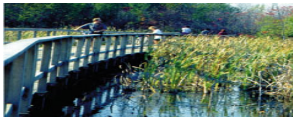
Figure 6: Example of a boardwalk crossing wetlands.
