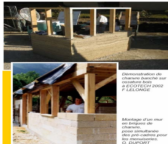
Figure 3: Timber frame and hemp brick walls.
