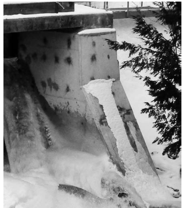
Dam pier with new cement cap, January 2009 Photos Ken Hook
