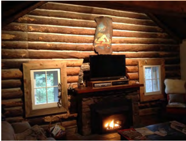
Stone fireplace with surrounding original wall, that was, at one time, hidden by paneling.
